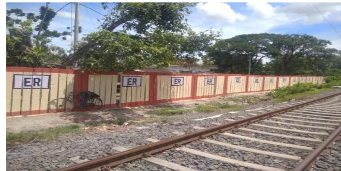
Boundary wall at Sealdah Division
