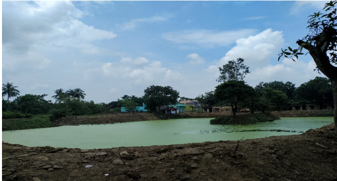
Rain Water Harvesting at Asansol Division
