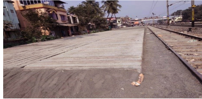
Approach road by using released PSCsleepers at Garifa /Howrah Division
