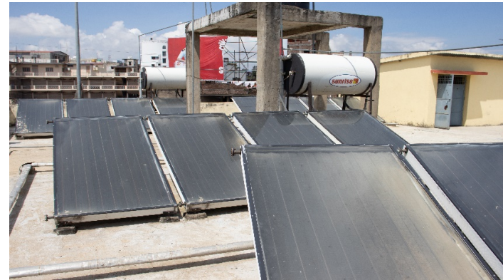
Solar Water Heater at Bhagalpur Station /ER
