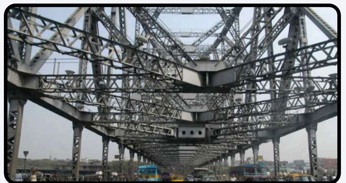
Close up structure of Howrah Bridge
