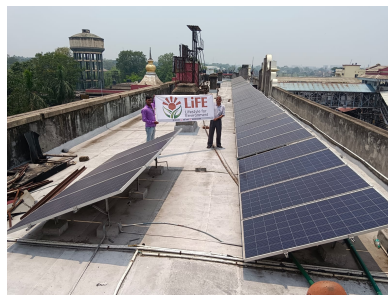
Asansol station building
