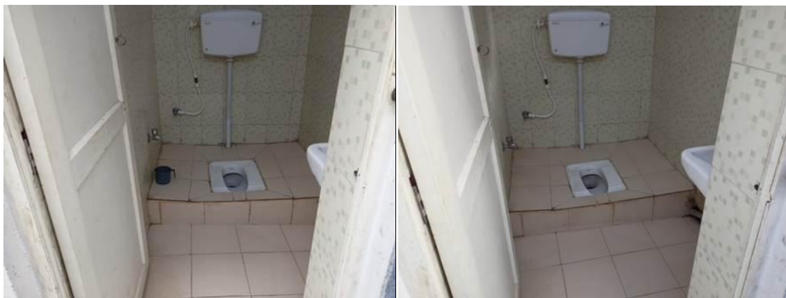
Before and after cleaning of Toilet at Health Unit Premises, BDC
