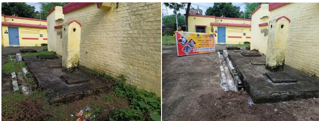
Before and after drainage cleaning of Septic tank at BDC Railway Colony
