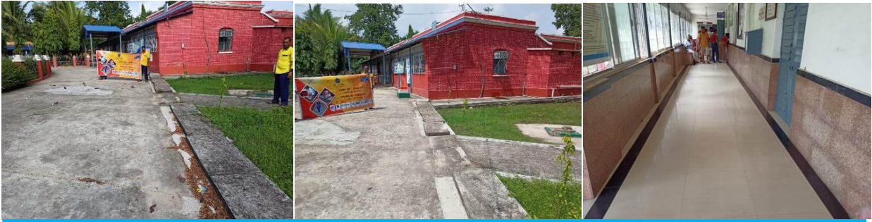
Before, during and after cleaning at Health Unit, BDC
