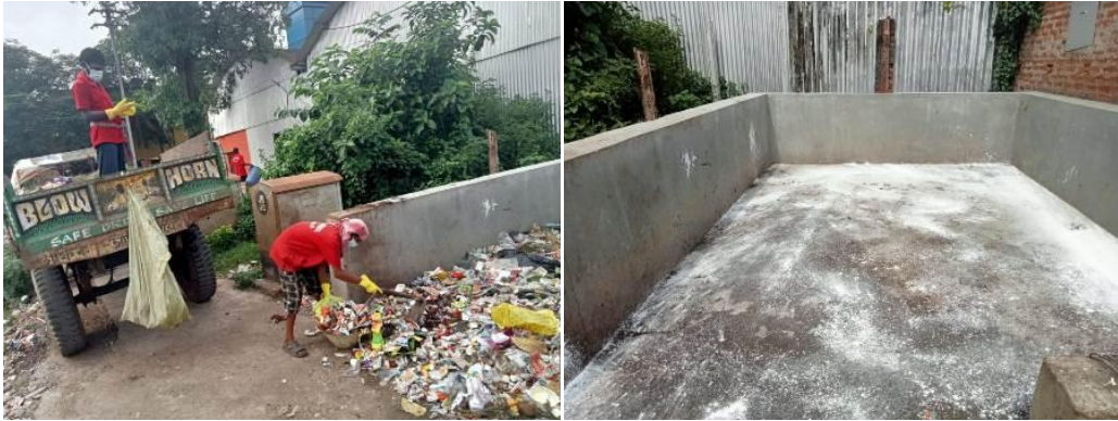
During and after Garbage Disposal at Railway New Colony, RPH
