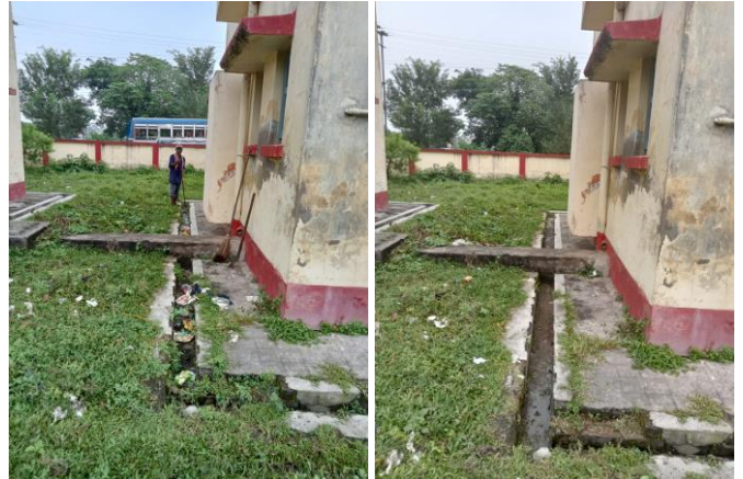
Drain cleaning at Panagarh
