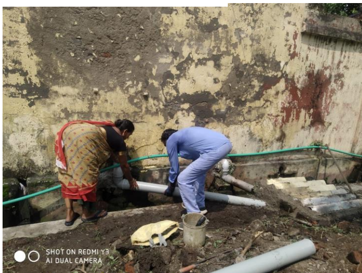
Sewer Line repair
