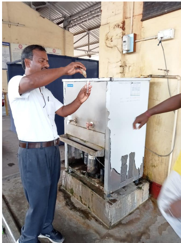
Residual Chlorine water testing, Health Unit, Panagarh
