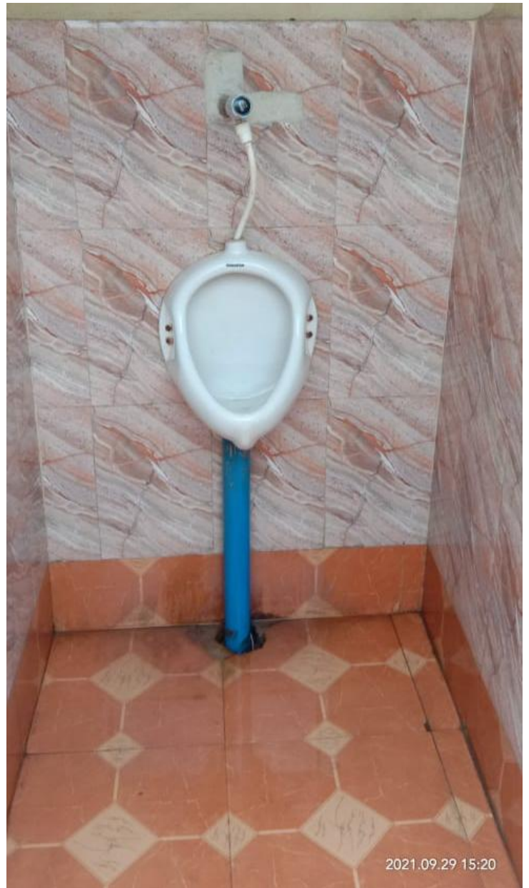
After Repairing Urinal Pipe at Panagarh Station
