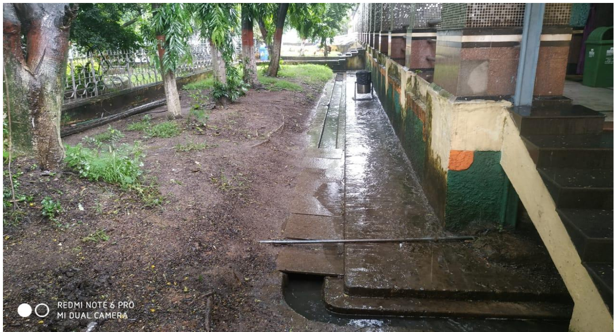
After Cleaning drain at Andal Station
