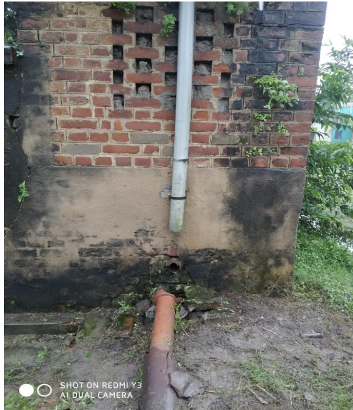
Before Repairing of Swere pipe line at Sitarampur Railway Colony
