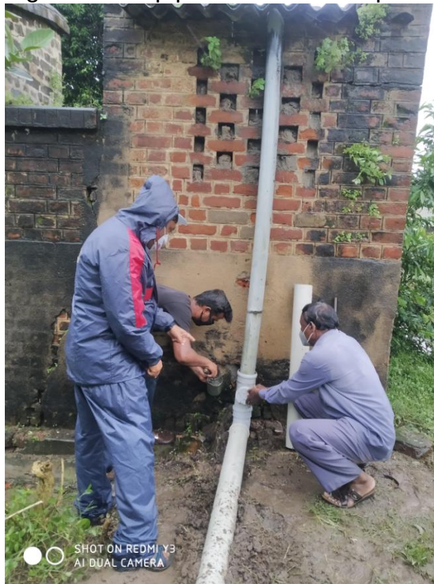
After Repairing of Swere pipe line at Sitarampur Railway Colony
