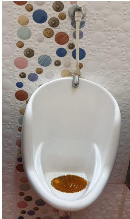
After cleaning of Urinal at Asansol Station
