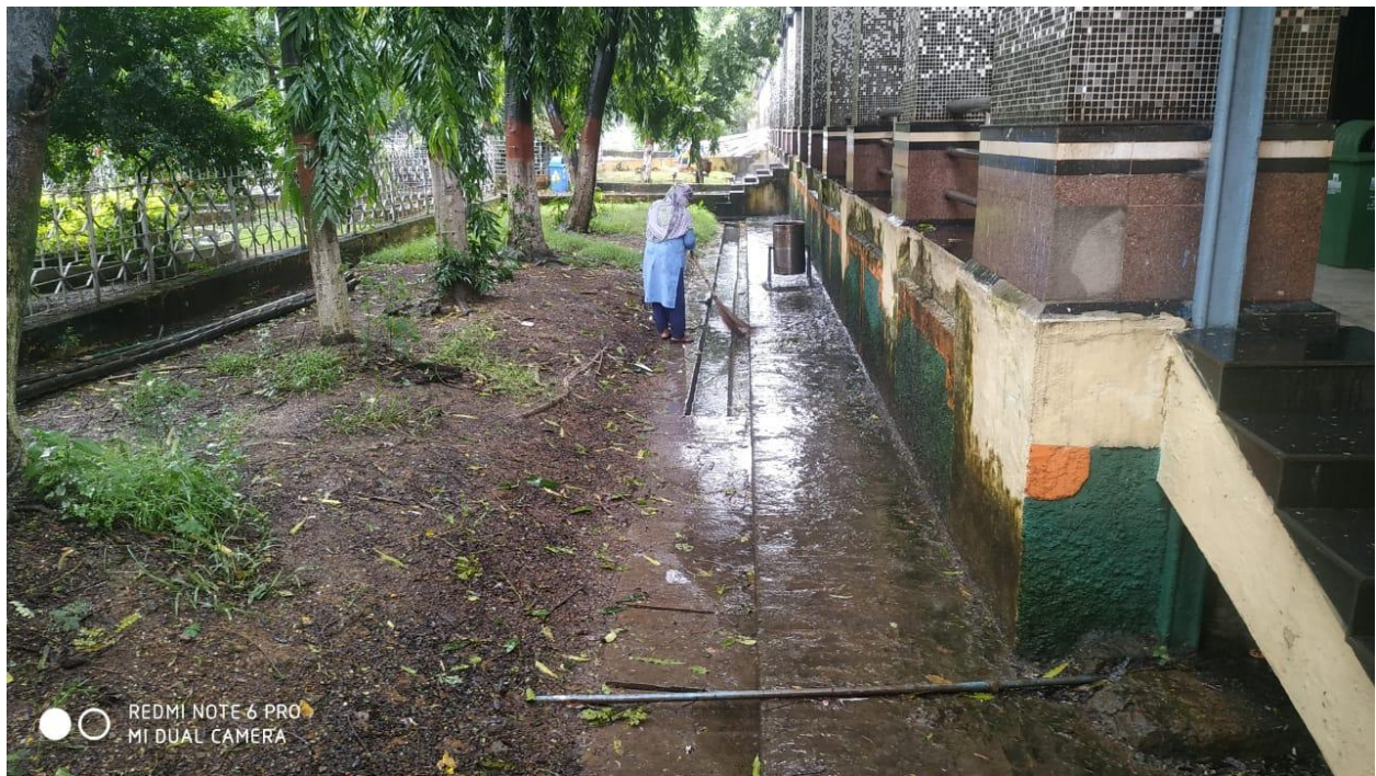
Before Cleaning drain at Andal Station
