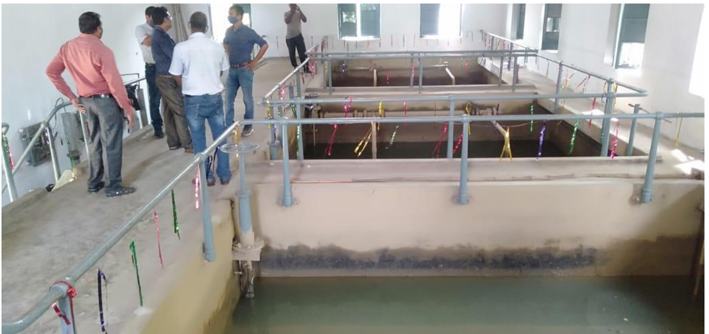
Inspection of Andal filter house and pump house near Damodar river by Sr.DEN III ASN
