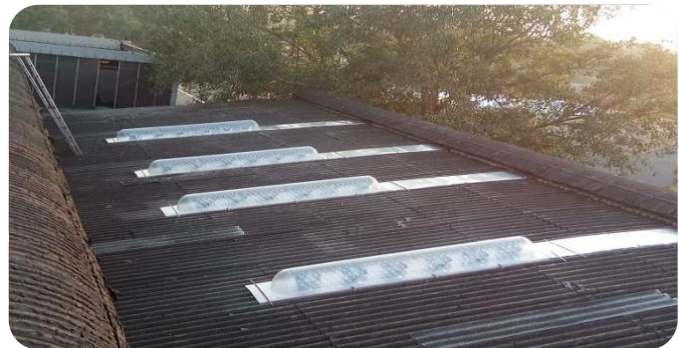
Solar Pipe Light installation on the roof of ELS/ASN
