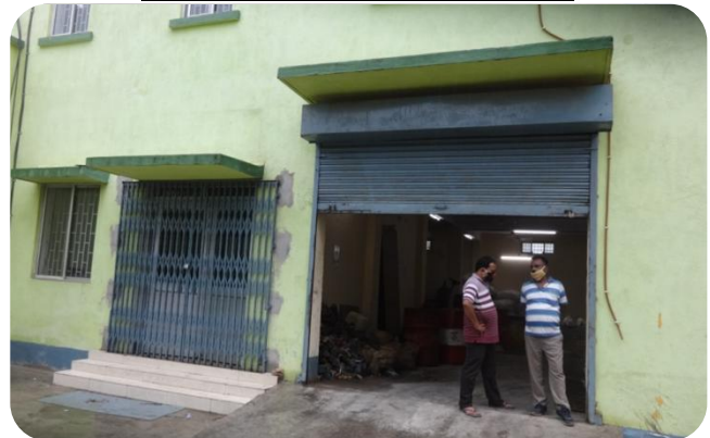
CAPITAL STORE BUILDING
