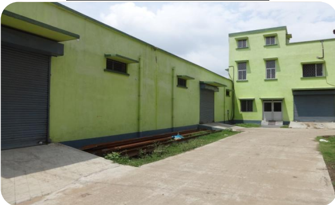
CAPITAL STORE BUILDING
