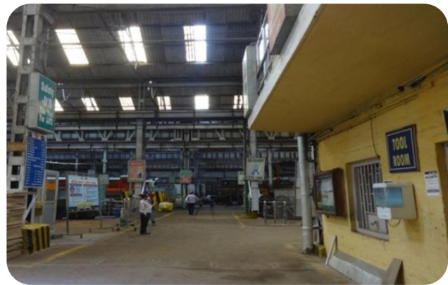
After installation of Solar pipe light
