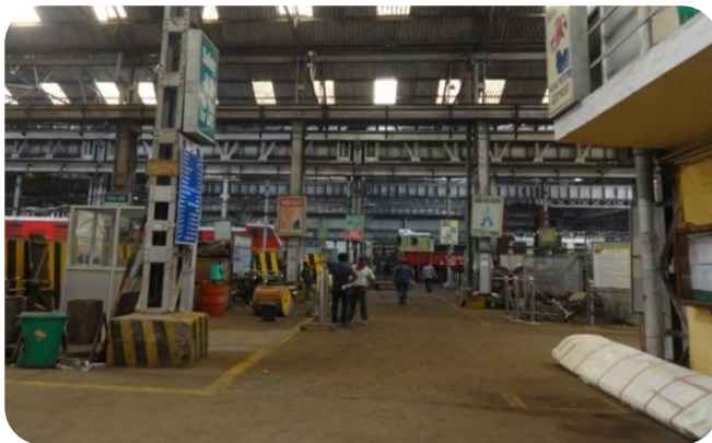
Before installation of Solar pipe
