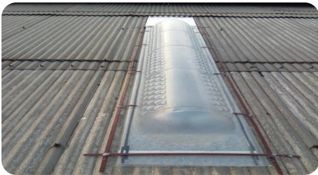
Solar Pipe Light installation on the roof of ELS/ASN
