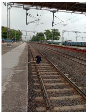
Before Cleaning of Railway track at RPNR on 28.09.2020
