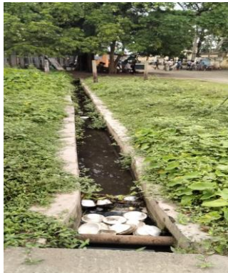
Before Cleaning of colony drain at Panagarh on 28.09.2020
