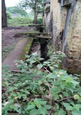
Before Cleaning of colony drain at Panagarh on 28.09.2020
