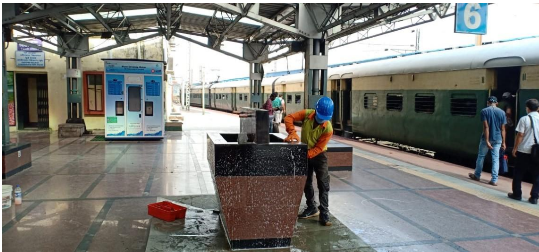
Before cleaning water booth at Asansol Station on 25.09.2020
