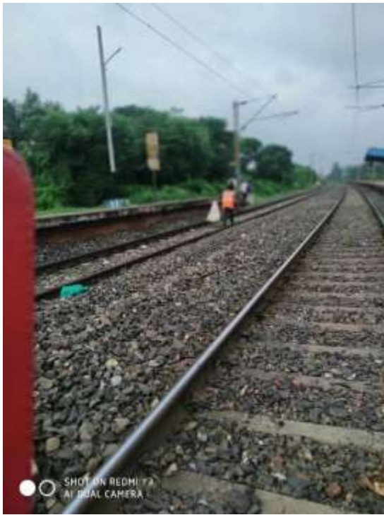
Before Cleaning of Railway track at Sitarampur Station on 26.09.2020
