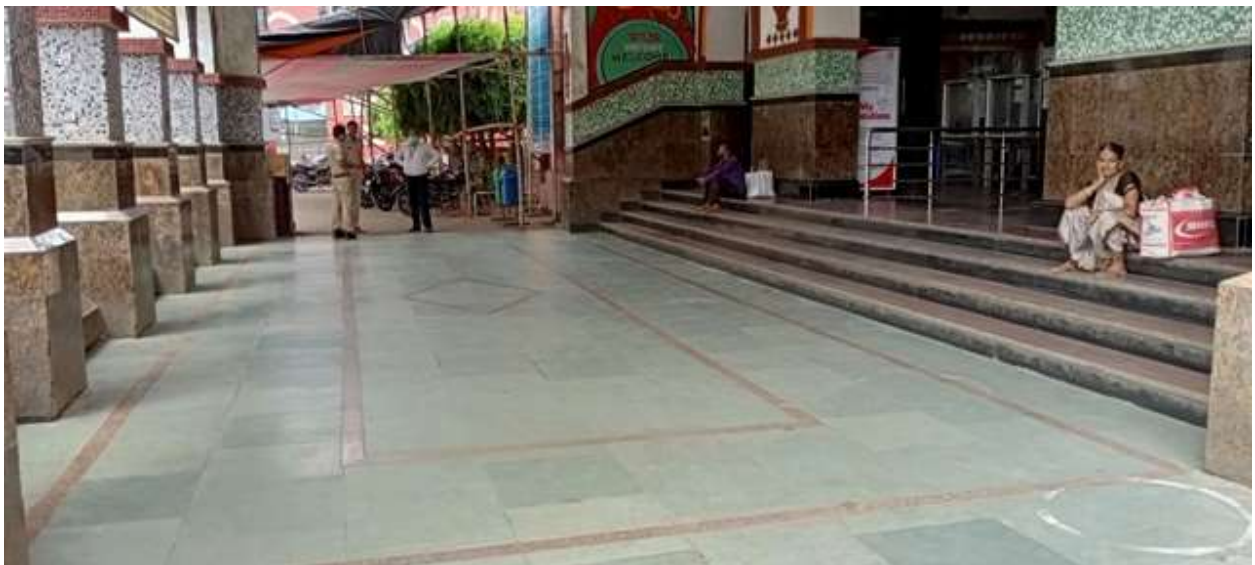
After cleaning of entrance Gate of Asansol Station on 26.09.2020
