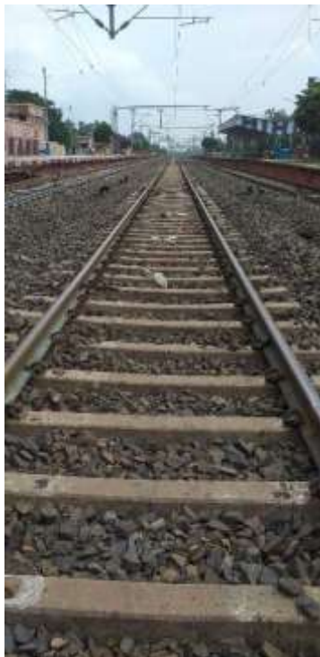
Before Cleaning of Railway track at Siuri Station-26.09.2020
