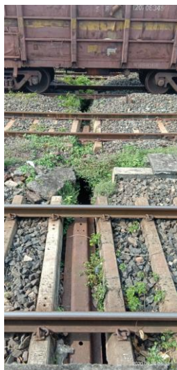
Before Cleaning of PF drain at Panagarh Station on 24.09.2020
