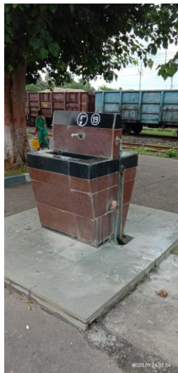
Before Cleaning of water booth at Panagarh Station on 24.09.2020
