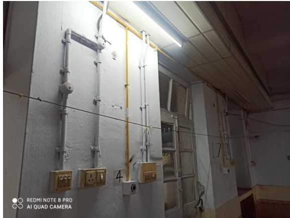
Ward being readied with Central Gas Pipeline
