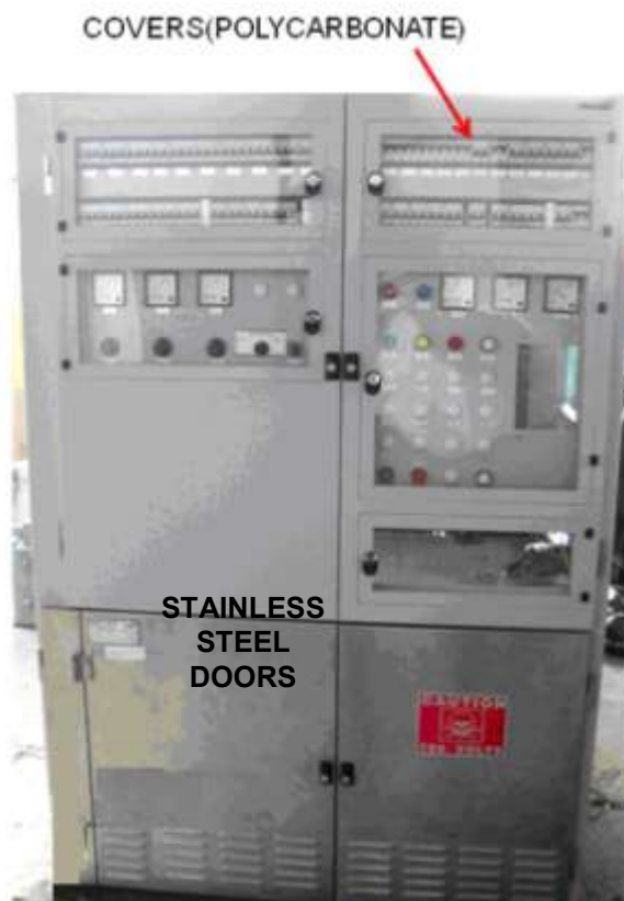
Figure 6.7 Modified Doors Arrangement
