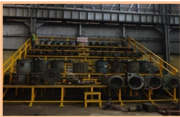
Auxiliary park before fitment of solar pipe lighting. Illumination=80 Lux.
