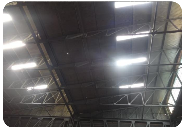
Commissioning of solar pipe lights / Day Light Harvesting
