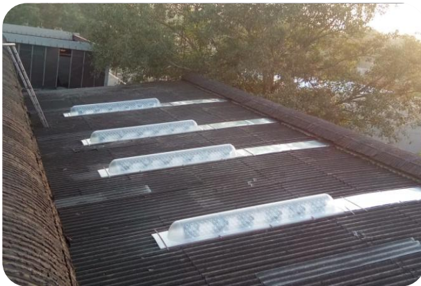
Commissioning of solar pipe lights / Day Light Harvesting
