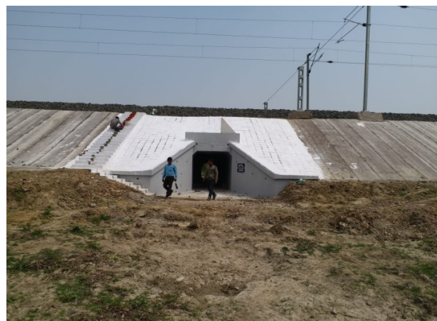
Bridge No.282 between Lalbag Court – Azimganj section
