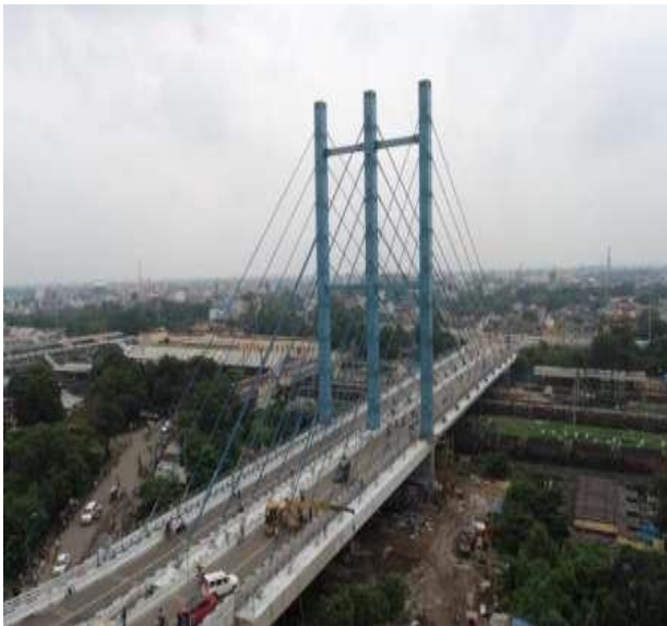
4 lane ROB at Barddhaman
