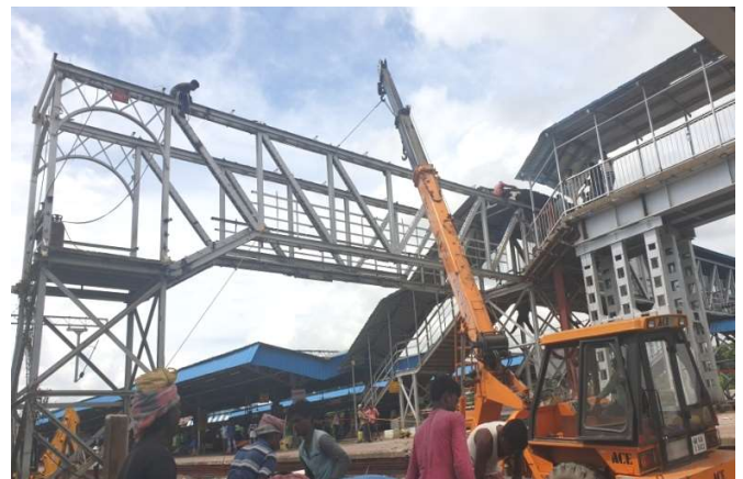
Dismantling & Commissioning of Extended FOB at MEMARI Railway Station
