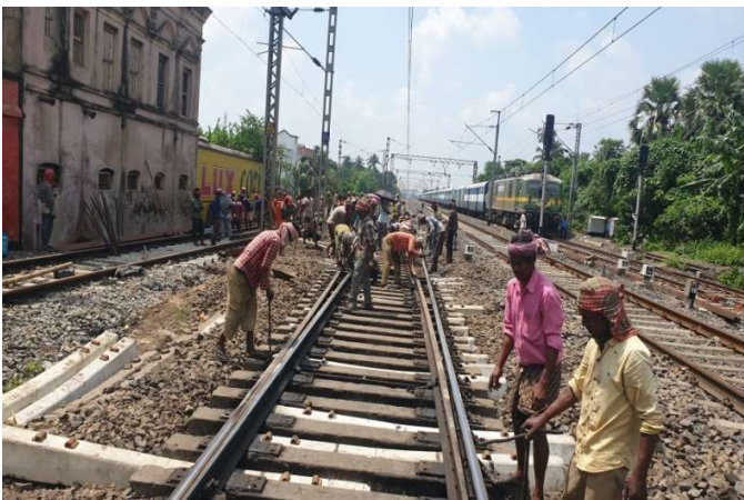
Yard Re-modeling at Rasulpur in connection with NI work of Debipur-Rasulpur 3 rd Line Work.
