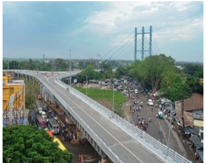
4 lane ROB at Barddhaman
