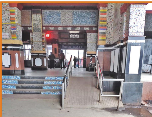
At Jamalpur Station
