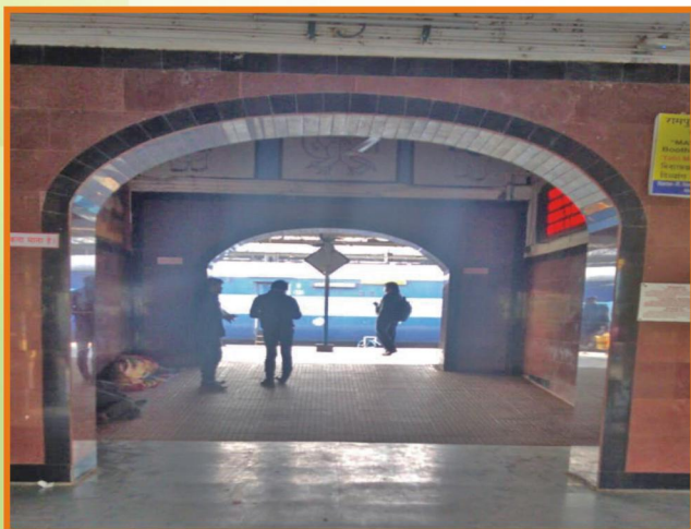
At Rampurhat Station
