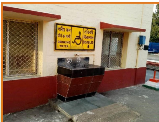
At Panagarh Station
