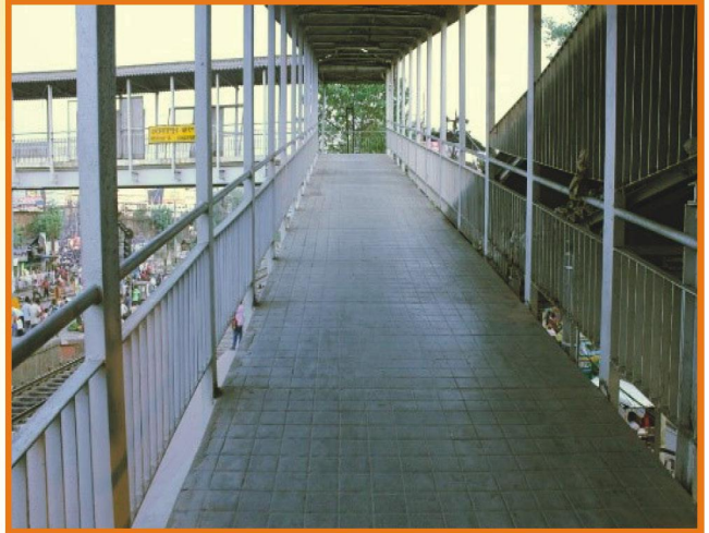
Ramp to Foot Over Bridge at Sonarpur
