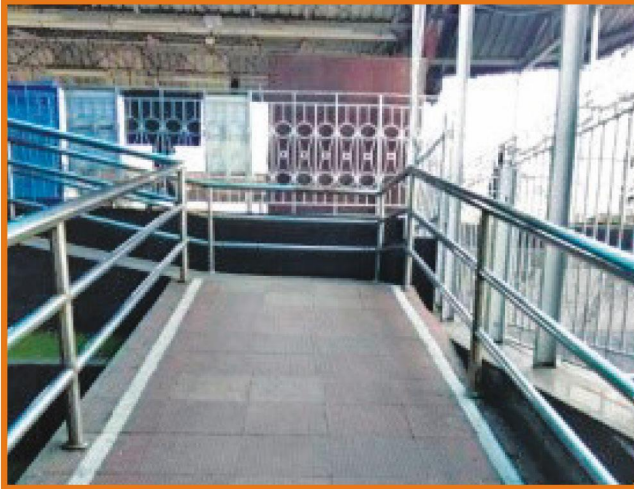
FOB ramp at Durgapur
