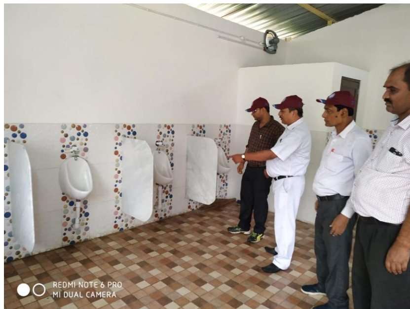
Inspection of toilet complex at Barakar station on 28.09.2019
