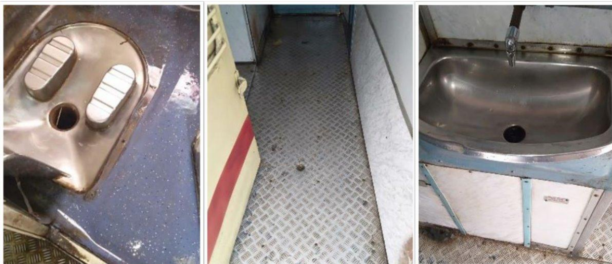
COACH CLEANING ACTIVITIES IN TRAIN No. 53523 AT ASANSOL OLD COACHING COMPLEX ON 25.09.19
