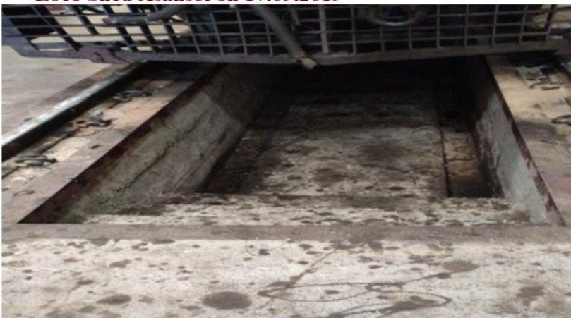
Before and after cleaning of inspection pit of Electric Loco Shed Asansol on 17.09.2019
