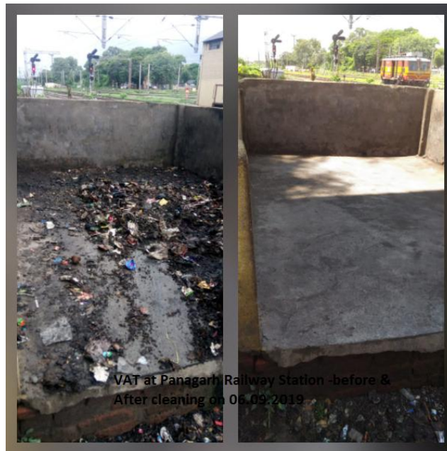
Before & After cleaning of VAT at Panagarh station
