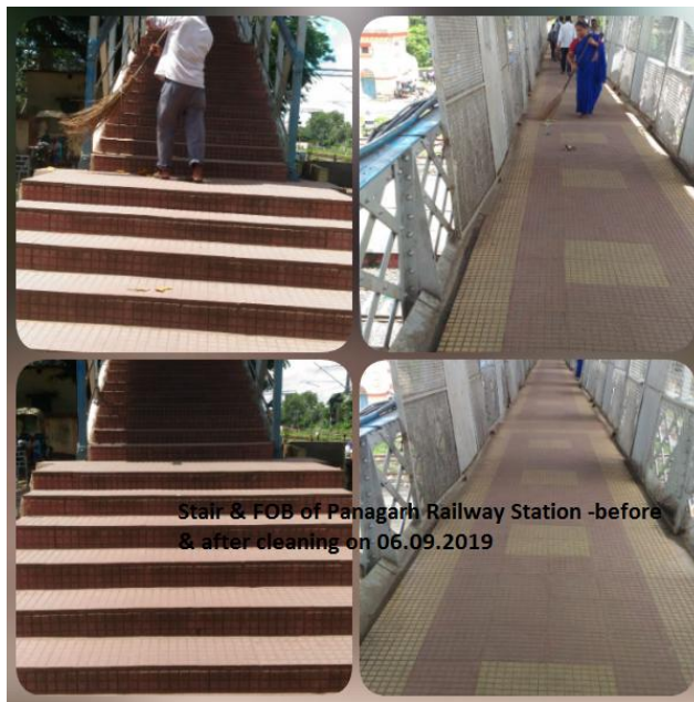
Before & after cleaning of Stair & FOB at Panagarh station
