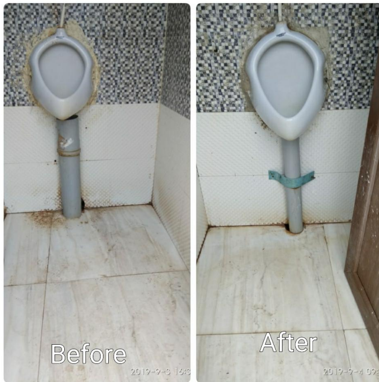
Before and after cleaning of Ladies toilet at Madhupur station on 04.09.2019
