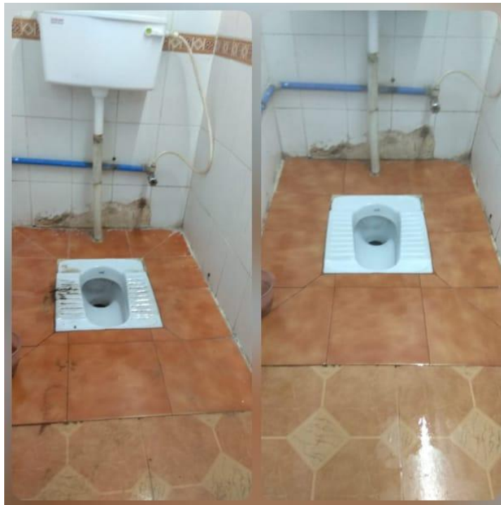
Before and after cleaning of Gents toilet at Durgapur station on 04.09.2019
