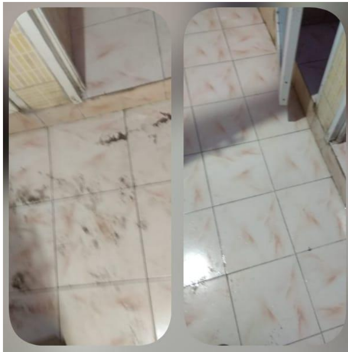
Before and after cleaning of Ladies toilet at Durgapur station on 04.09.2019
