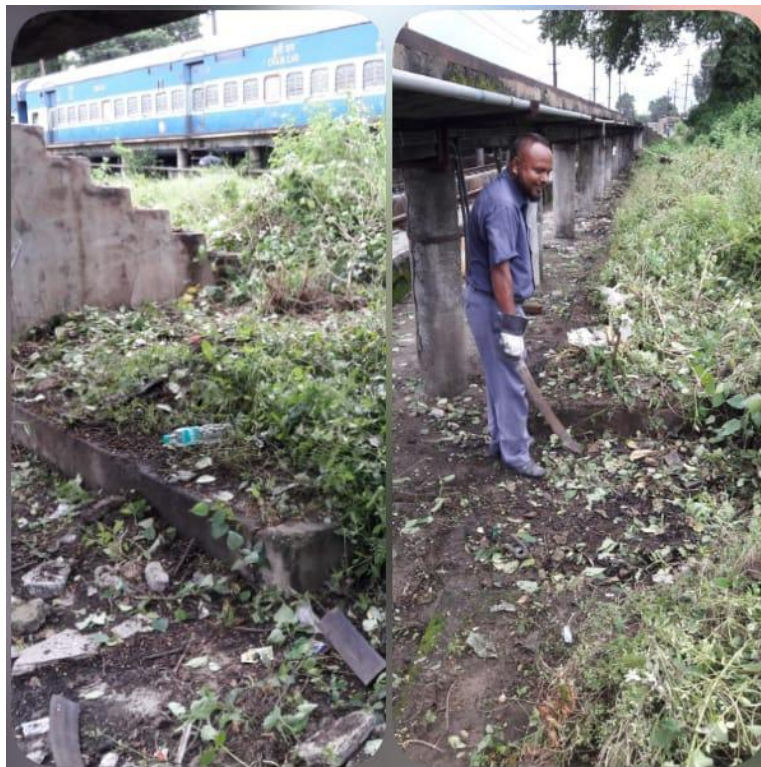
Before and after cleaning of Old Coaching Complex Asansol on 04.09.2019
