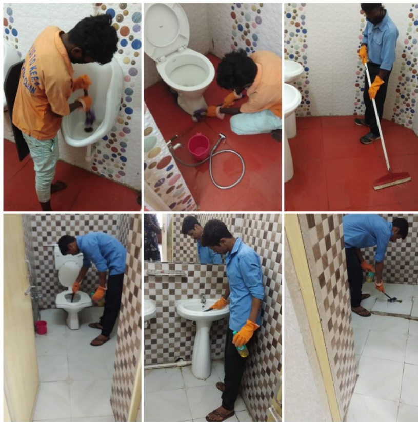
Before cleaning of Premium lounge at Asansol Station on 03.09.2019
