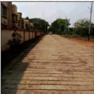
The road is made from disposable released concrete sleepers
