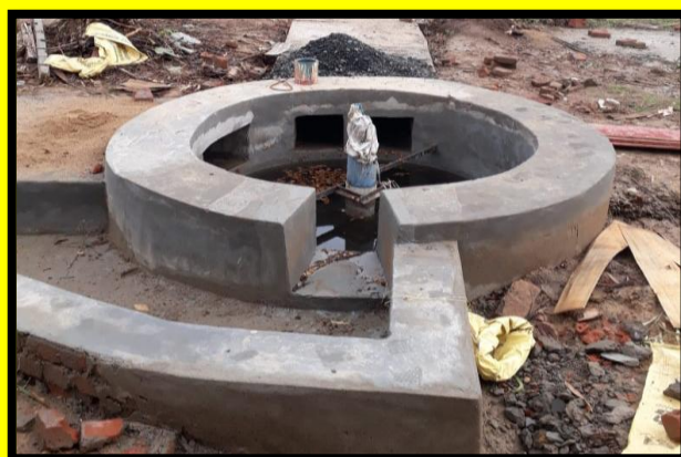
Rain Water Harvesting Arrangement in Asansol Hospital
