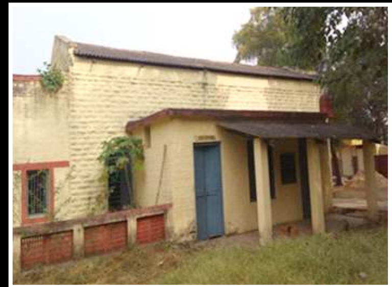
Kalubathan Station Building
