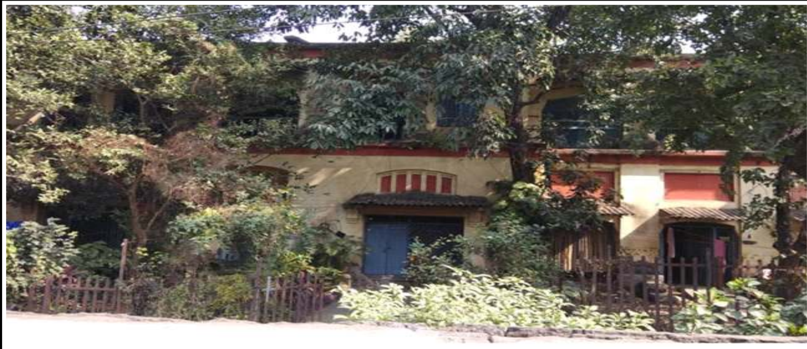
Heritage Structure of Old DS's Bungalow-cum-Office
