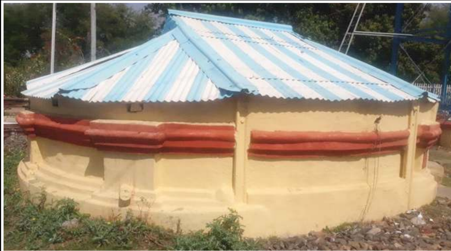
Heritage Structure of Madhupur Well
