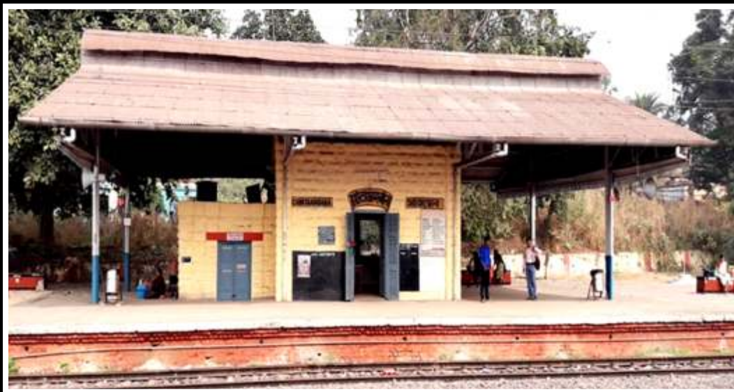
Chota Ambana Station Building
