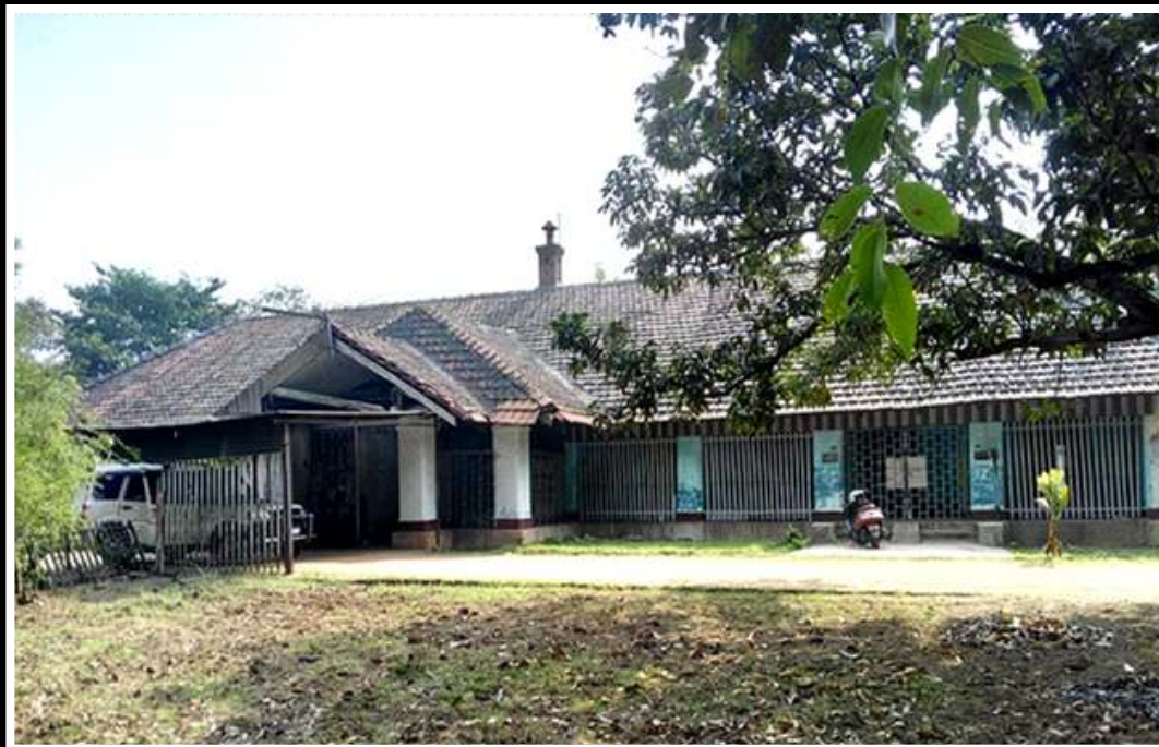
Heritage Structure of Old DS's Bungalow/ROTC
