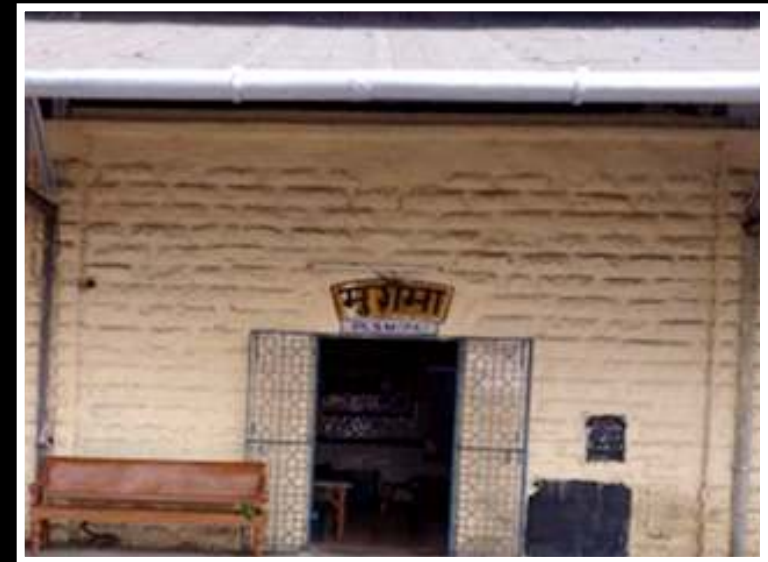
Mugma Station Building
