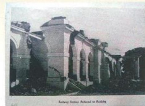
Railway Station Reduced to Rubble
