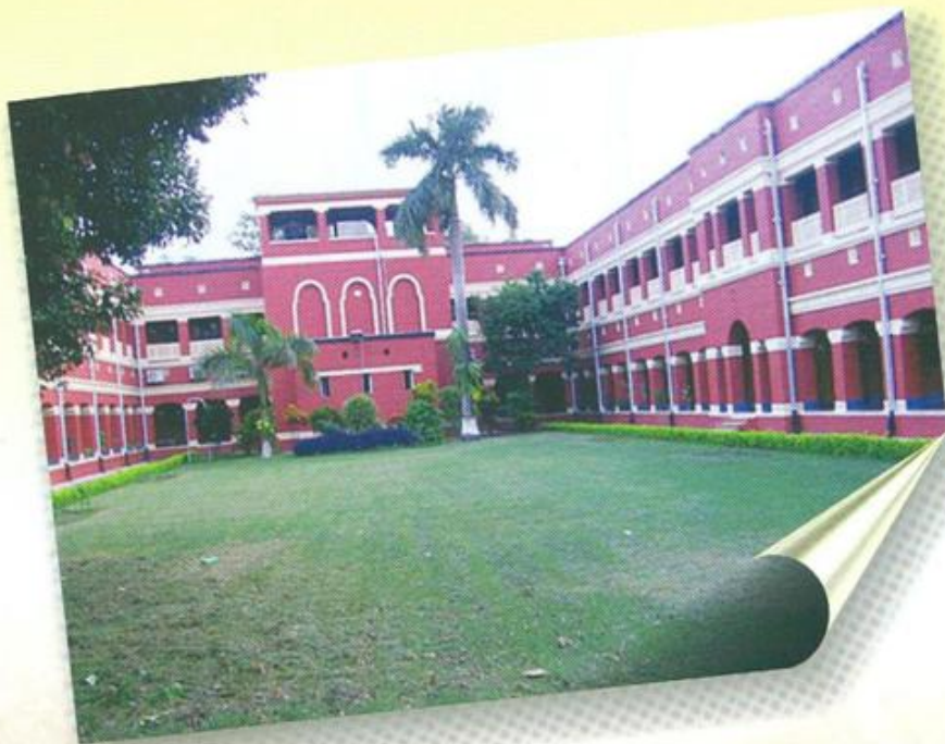
View of Gymkhana from Quadrangle
