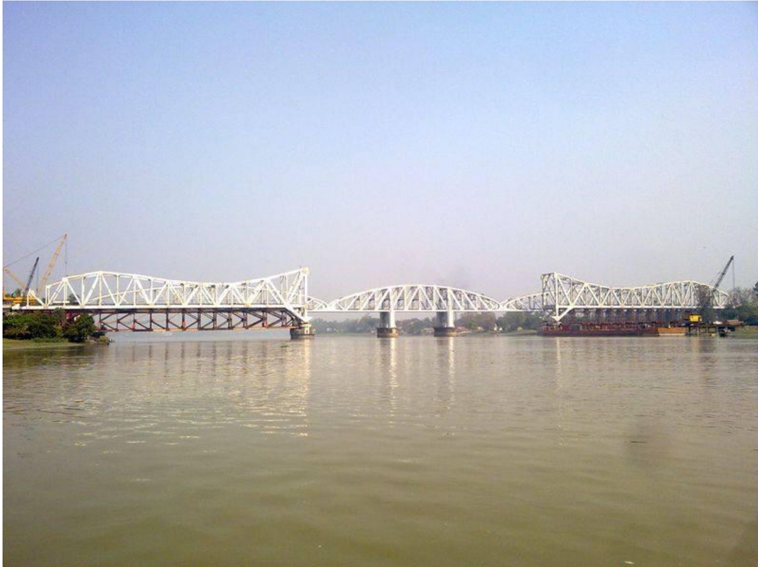
Erection in new Jubilee Bridge in Progress in foreground. Old Bridge in background.
