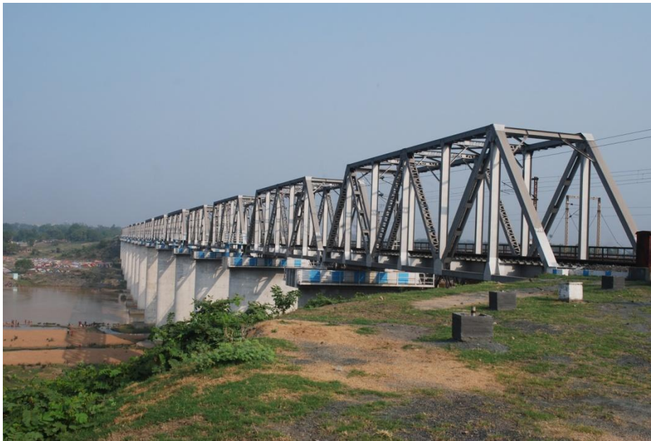
Newly commissioned Barakar Bridge (22.07.14)
