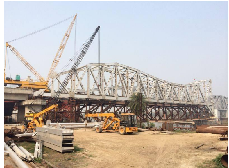
Bandel end being erected
