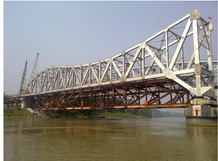
Bandel end span erected
