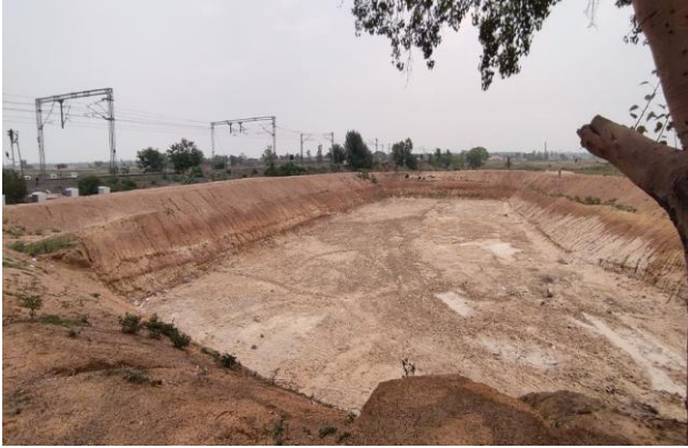
Artificial pond at Pandaveshwar for Rain water harvesting
