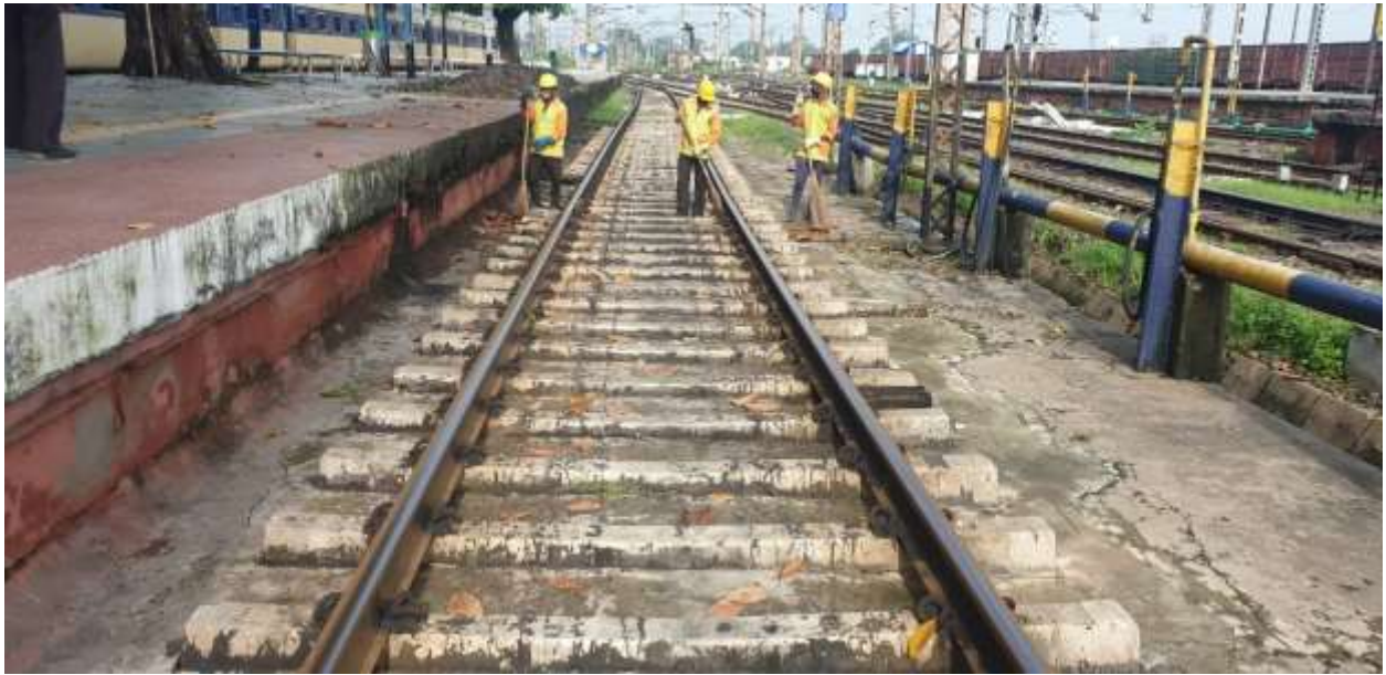
Before cleaning the Railway track at Asansol on 27.09.2020
