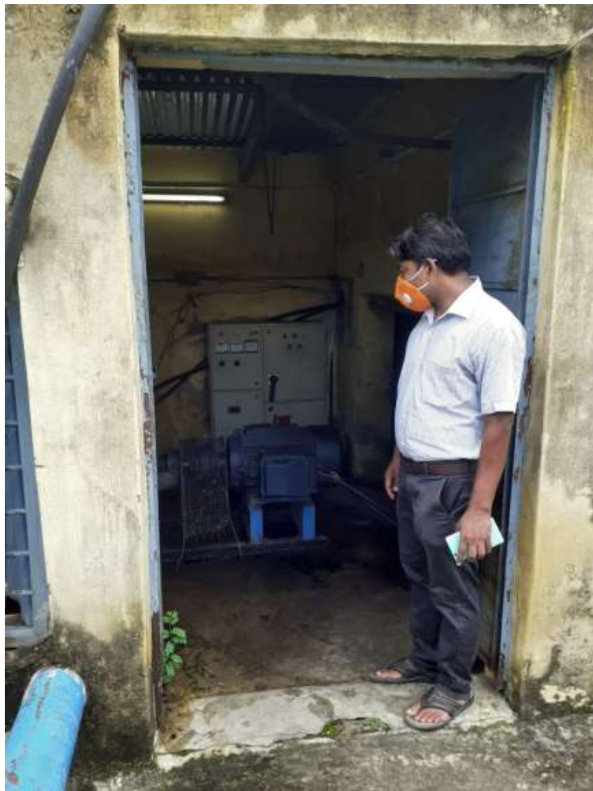
Inspection of pump house at Andal on 19.09.2020
