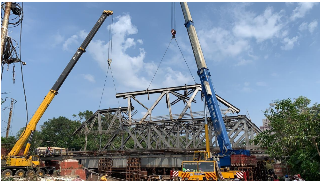
DISMANTLING OF FIRST TRUSS BY 2 NO.S 150 T ROAD CRANE
