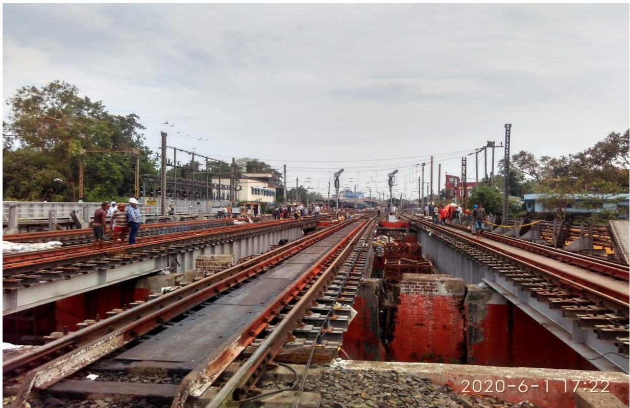
BRIDGE 1 AFTER DISMANTLING OF OLD REDUNDANT TRUSS
