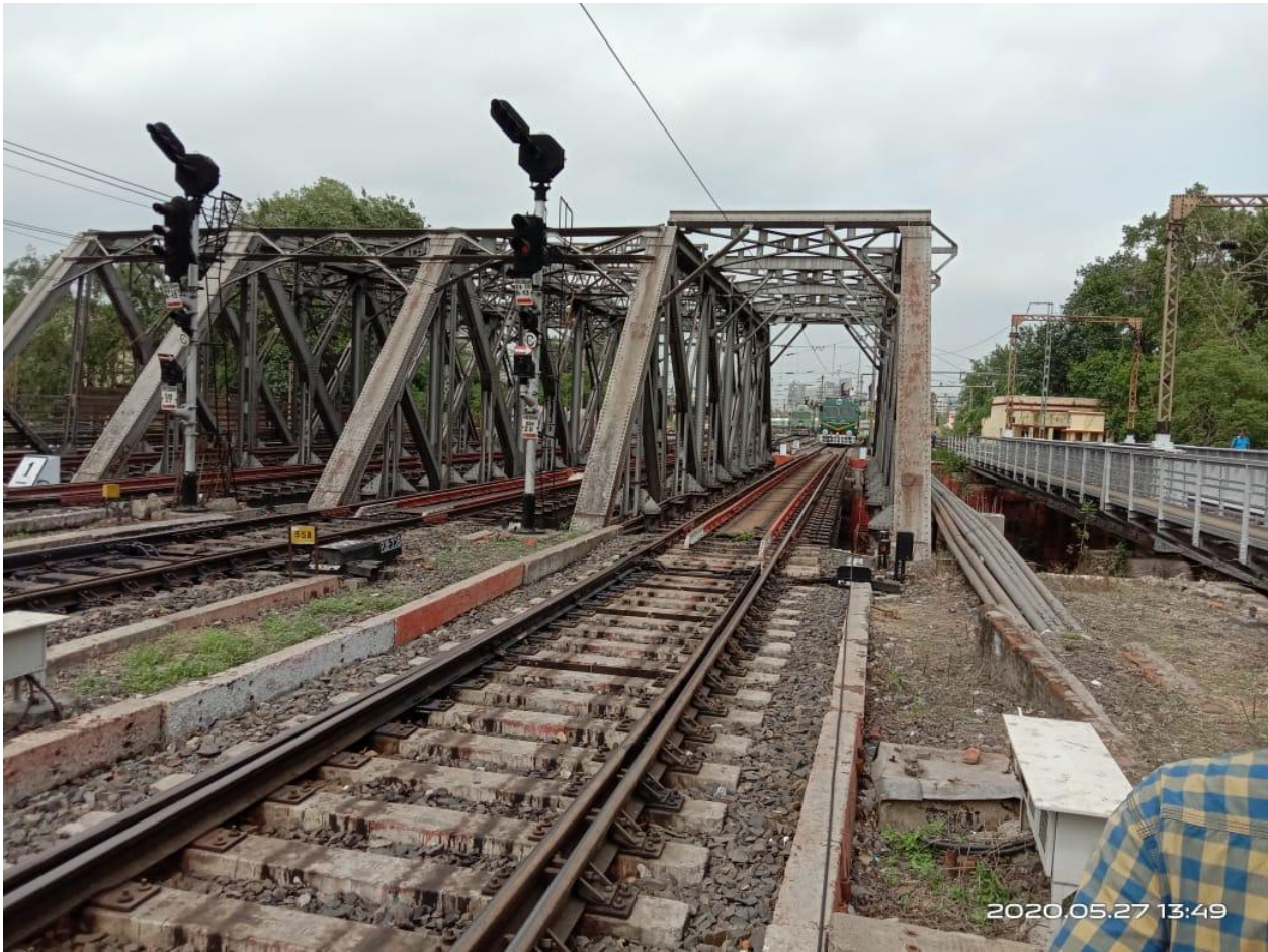
BRIDGE 1 PRIOR TO DISMANTLING
