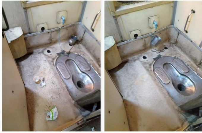
CTS ACTIVITIES IN TRAIN No. 12322 ON 29.09.19 AT ASANSOL
