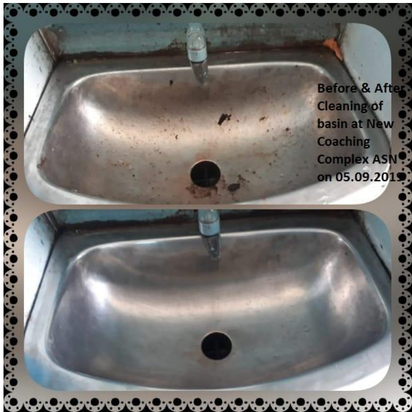
Cleaning at New Coaching Complex Asansol on 05.09.2019
