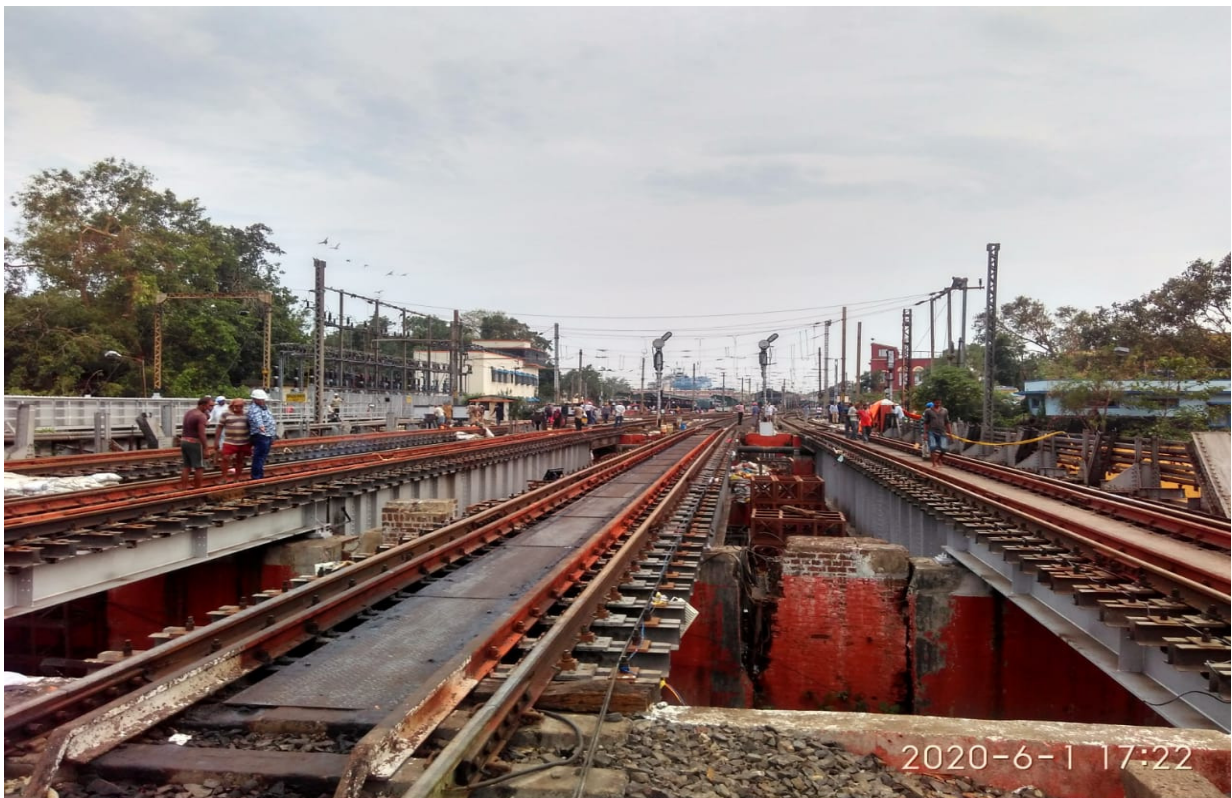
BRIDGE 1 AFTER DISMANTLING OF OLD REDUNDANT TRUSS
